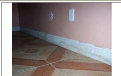
baseboard in laundry room
